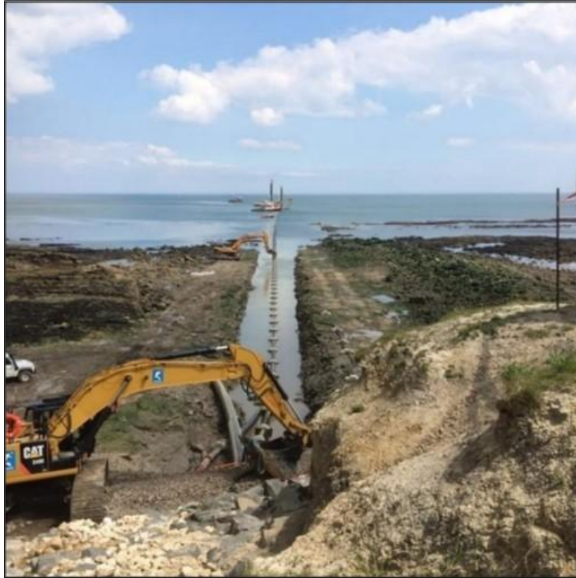
Figure 5-4: Photo showing installation of a cable in a trench at a landfall.
