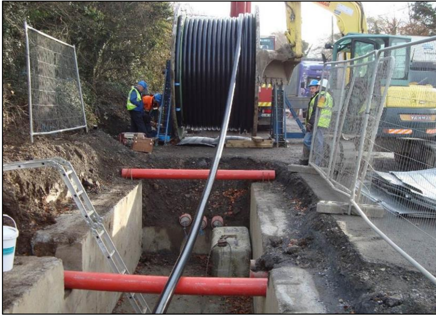
Figure 5-5: Photo of cable pulling procedure.
